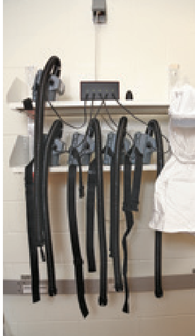
Air purifying respirators, part of the protective equipment worn in the presence of possible infectious agents.
