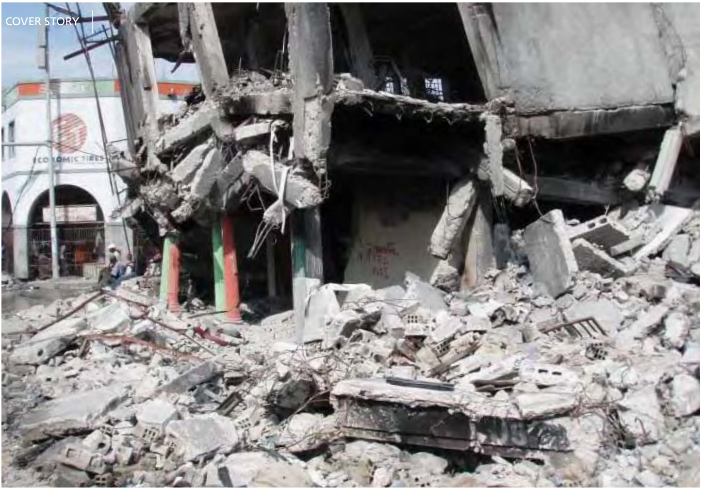
Crumbled buildings like this were common in downtown Port au Prince following the massive earthquake.
